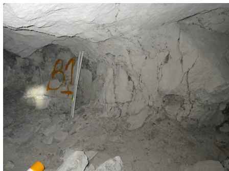
Figure 6—Photo of pillar B, side 1
