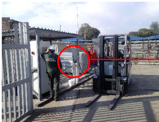
50-200 bar 13 Nm 3 H 2 /h MH H 2 compressor integrated in hydrogen refuelling station
