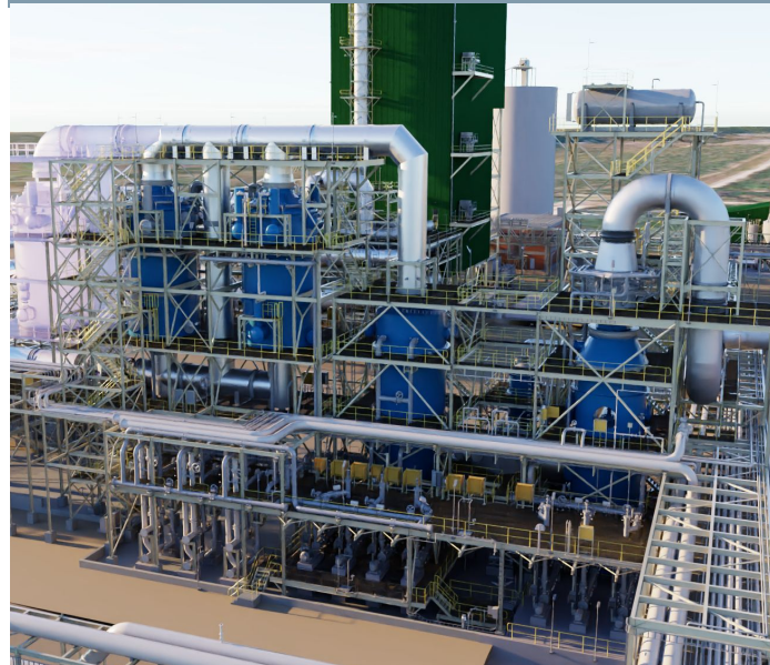
Wet Gas Cleaning Plant
