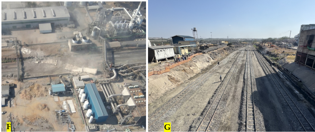
Figure 7: Cleaning progress area after converter stack demolition where in F (cleaning ongoing) and G (cleaning completed) ( https://dracogroup.co.za , 2026).
