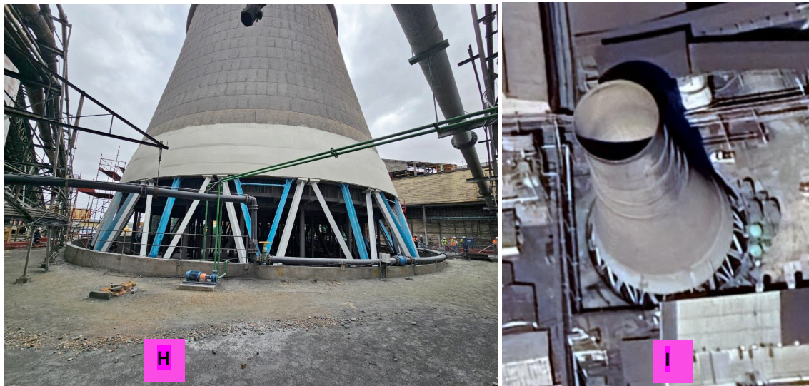
Fig. 9: View of the PMC smelter hyperbolic cooling tower (H) immediately after rehabilitation in 2024 and (I) from Google Earth (2026).
