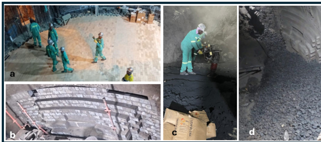
Figure 16: (a) Alumina brick installation on the hearth; (b) completed V-shape installation; (c) carbon ramming installation; (d) electrode paste cubes loaded onto hearth.
