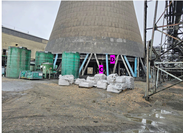
Fig. 7: Rehabilitation of the PMC smelter cooling tower involving change of concrete beams (C) to steel beams (D).
