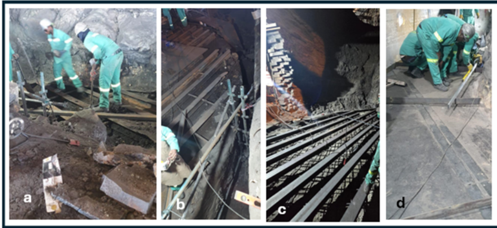
Figure 14: (a) Cleaning metal and debris between grillage beams; (b) and (c) new grillage beam installation; (d) new bottom plate sections and level checks.
