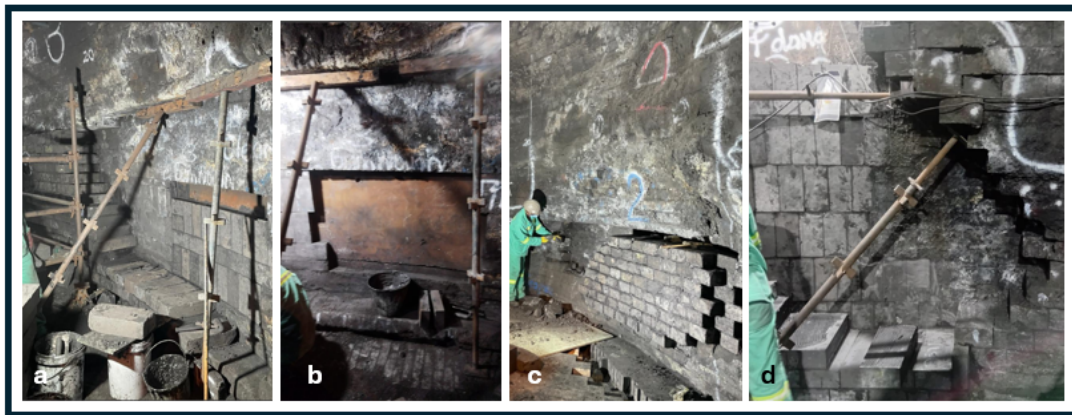
Figure 15: (a) Supports being put to hold the clover sidewall while installing new carbon bricks; (b) Damaged tiles are taken off the shell while the area is being supported; (c) building below the metal line at a clover; (d) Scaffold pipe supports put in place prior to removing and building bricks underneath a sidewall.
