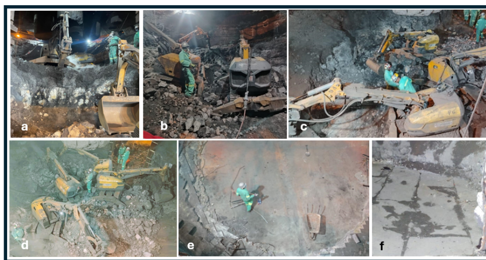
Figure 13: (a) Breaking chrome at the entrance of furnace; (b and (c)) multiple brokks focusing on chrome breaking below the electrodes; (d) multiple brokks with buckets and moils focusing on opening up the areas in front of the sidewalls; (e) demolition complete to show bottom plate; (f) damaged bottom plates to be replaced.
