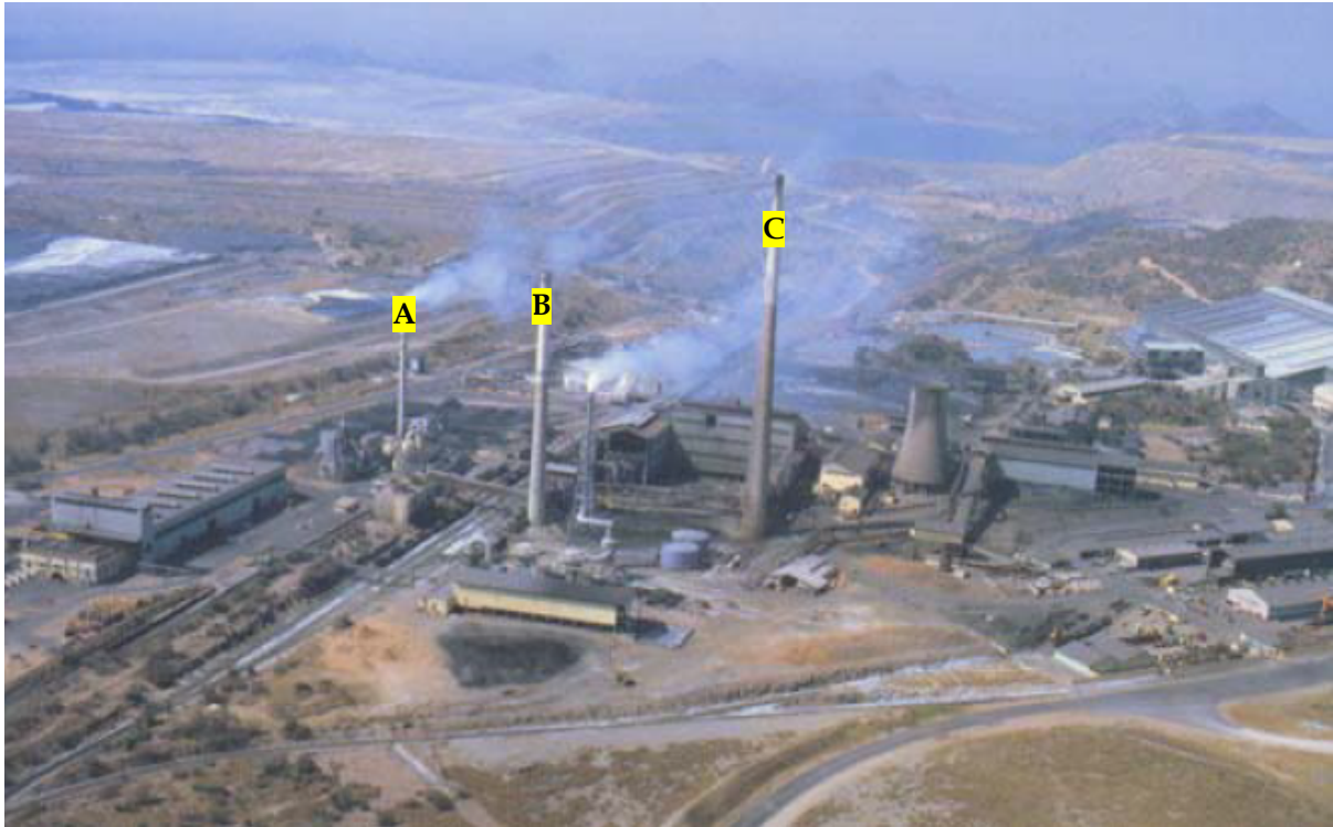
Figure 5: PMC smelter with three stacks: A – acid plant i.e., 75 m; B – converter i.e., 107 m and C – reverberatory i.e., 154 m (Jones and Mackey, 2015).
