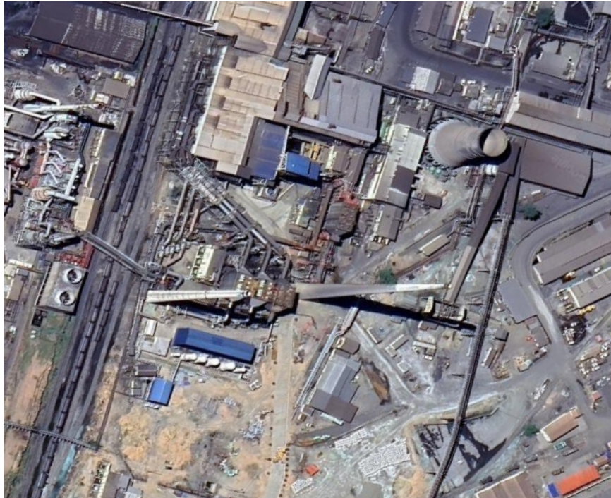
Figure 8: PMC smelter area after the demolition of the converter stack ( https://earth.google.com , 2026).
