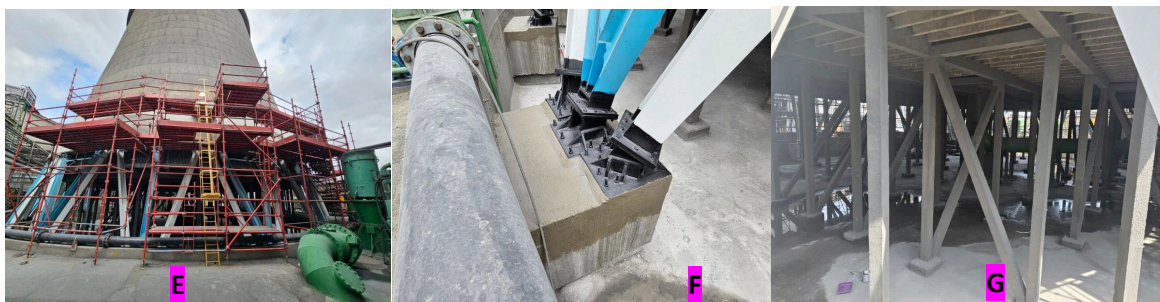
Fig. 8: Final rehabilitation involving changing all remaining concrete to steel beams (E), enlargement of plinths to accommodate steel knuckle bases (F) and refurbishment of internal pond columns (G).
