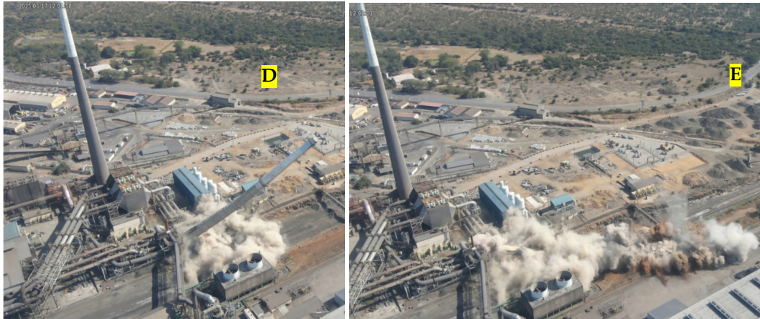
Figure 6: Converter stack demolition in D and E during June 2025 ( https://dracogroup.co.za , 2026).
