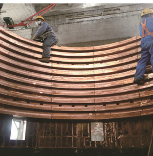
铅冶炼侧吹炉铜水套现场安装照片 photo of copper water jacket installation in lead smelting side blow furnace
