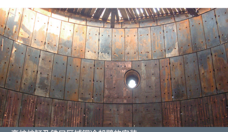
高炉炉缸及铁口区域铜冷却壁的安装 hearth and iron taphole area copper stave installation in blast furnace
