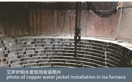
铜冶炼侧吹炉铜水套现场安装照片 photo of copper water jacket installation in side blow furnace
