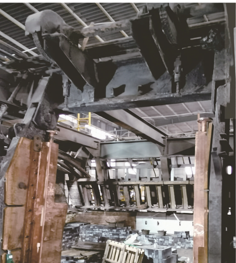
倾动炉铜水套现场安装照片 photo of copper water jacket installation in tilting furnace
