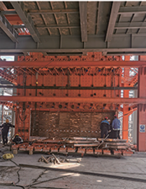
烟化炉铜水套现场安装照片 photo of copper water jacket installation in fuming furnace
