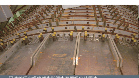
闪速炉反应塔底部齿形铜水套现场安装照片 photo of toothed copper water jacket installation at the bottom of the flash furnace reactor
