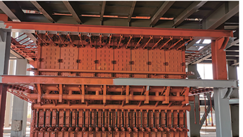
烟化炉铜水套现场安装照片 photo of copper water jacket installation in fuming furnace
