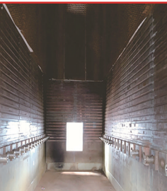
烟化炉铜水套现场安装照片 photo of copper water jacket installation in fuming furnace
