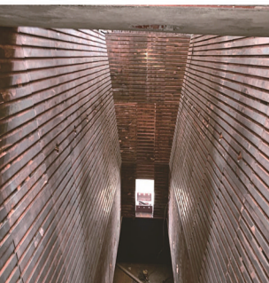
铜冶炼侧吹炉铜水套现场安装照片 photo of copper water jacket installation in side blow furnace
