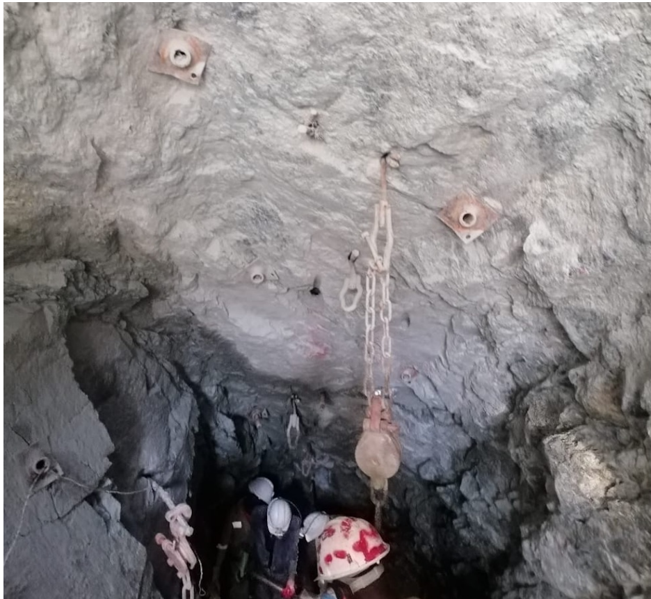
Figure 2: Example of Split Set Installation in Winze
