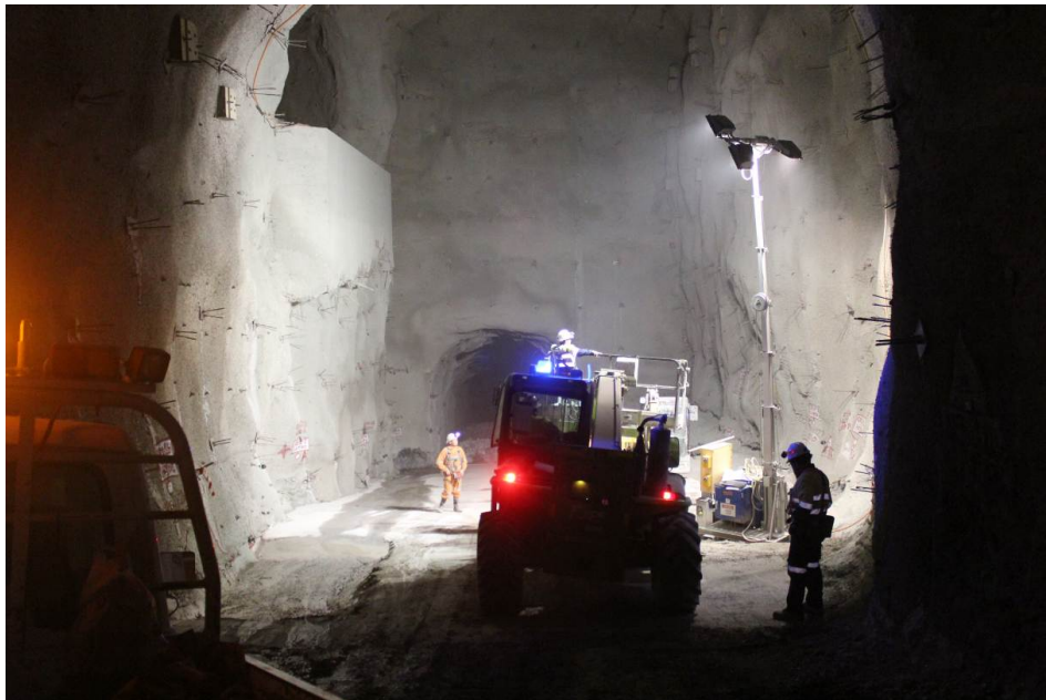
Figure 11: Shotcrete application Cadia East mine, NSW Australia.
