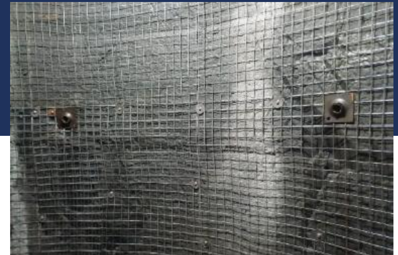
Image: Mesh and bolting of sidewall.
