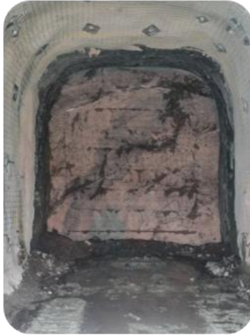
MC51 Underground – Cutting Face
