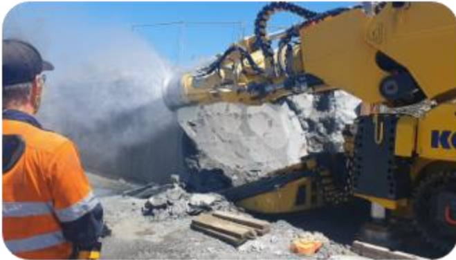
Factory Acceptance Testing Before Deployment
