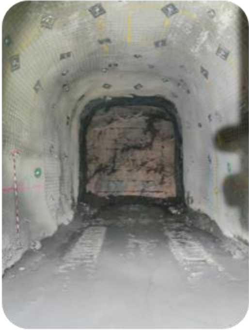
MC51 Underground – Cut Tunnel with Ground Support
