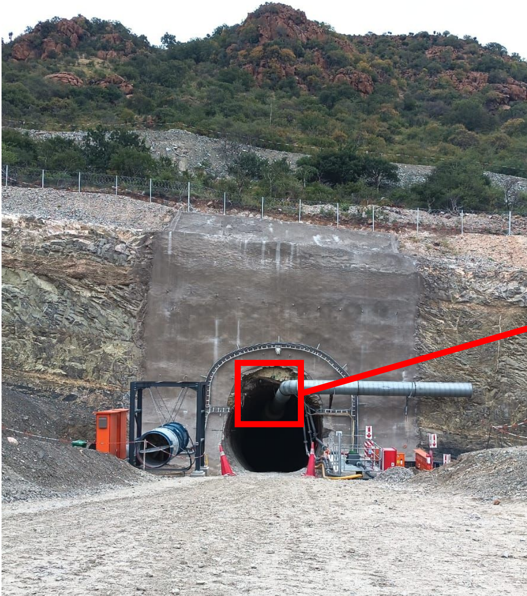
Image 16 : MTB portal entrance, challenging ground conditions
