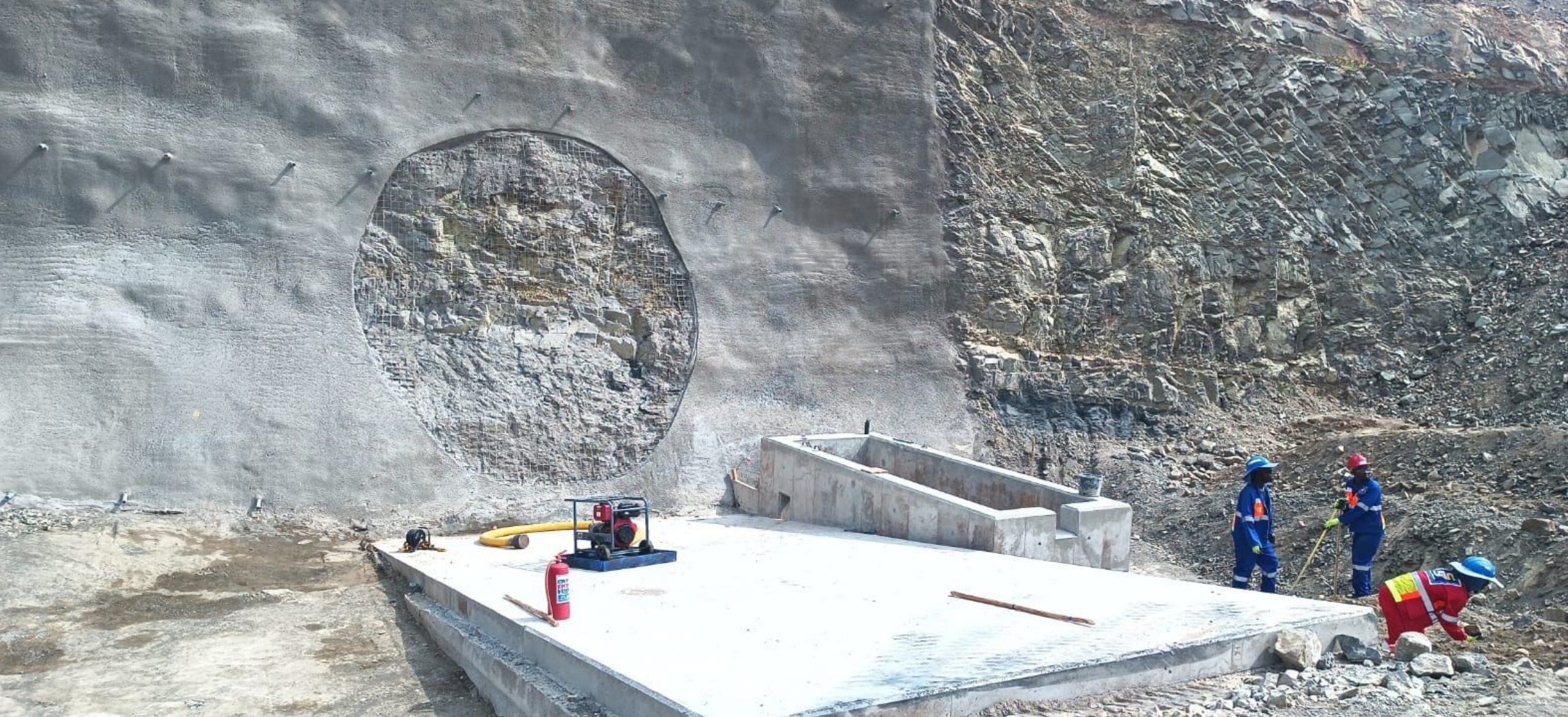
Image 11: MTB launch pad at portal – showing -9° dip
