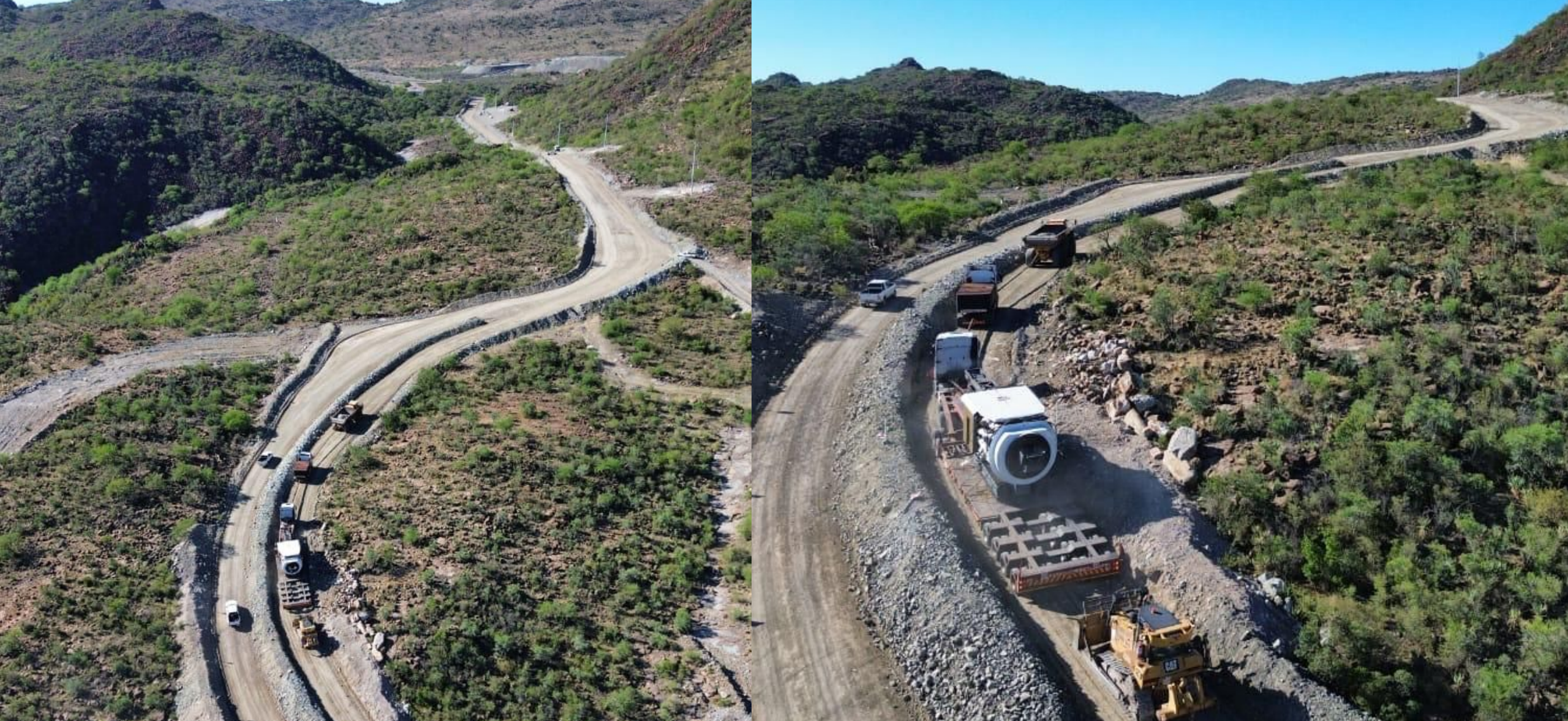
Image 9 & 10: Transportation of MTB to site
