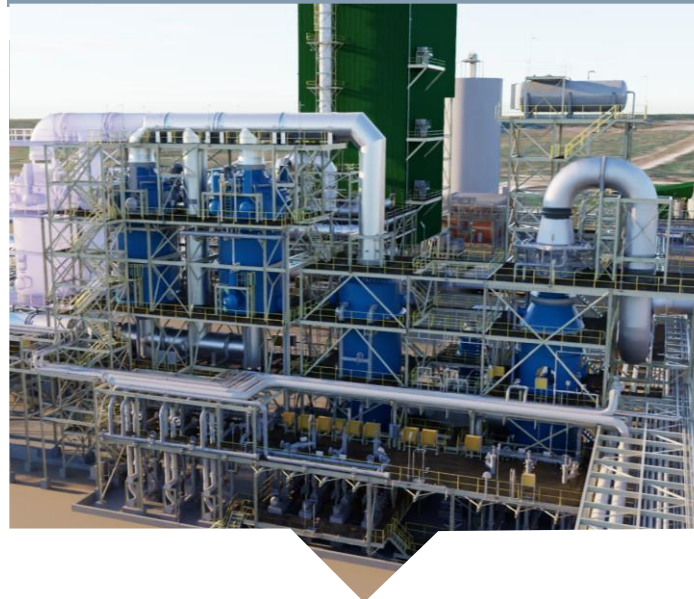
Wet Gas Cleaning Plant
