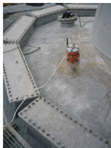
View of Tower Top Demister Panel Access Doors
