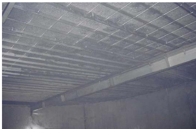
View from below of a Drying Tower Demister
