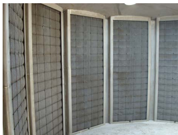
Inside View of Vertical Demister Panel Polygon
