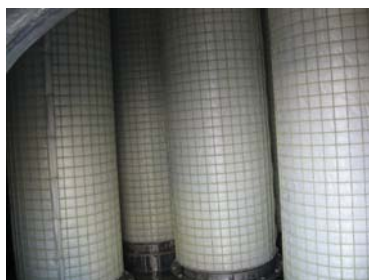
B14W Glass Rope Standing Candle Filters
