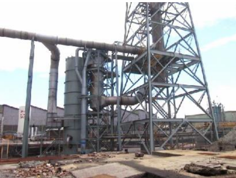
Port Kembla Copper Tail Gas Scrubber Installation
