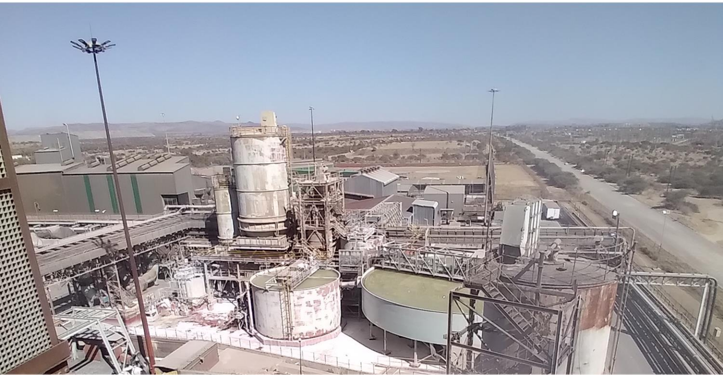
Marikana Smelter Dual Alkali Regeneration System
