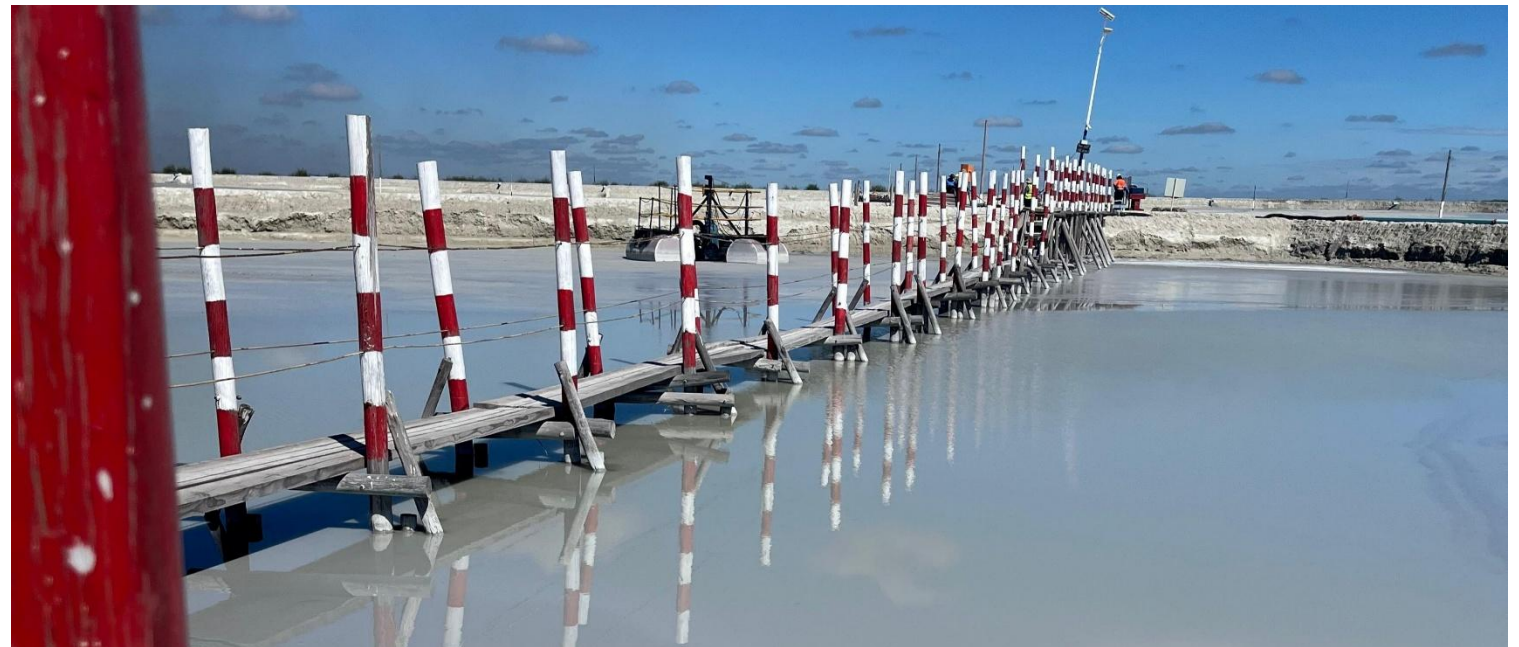
Photo: SRK archives - timber catwalk on platinum TSF
