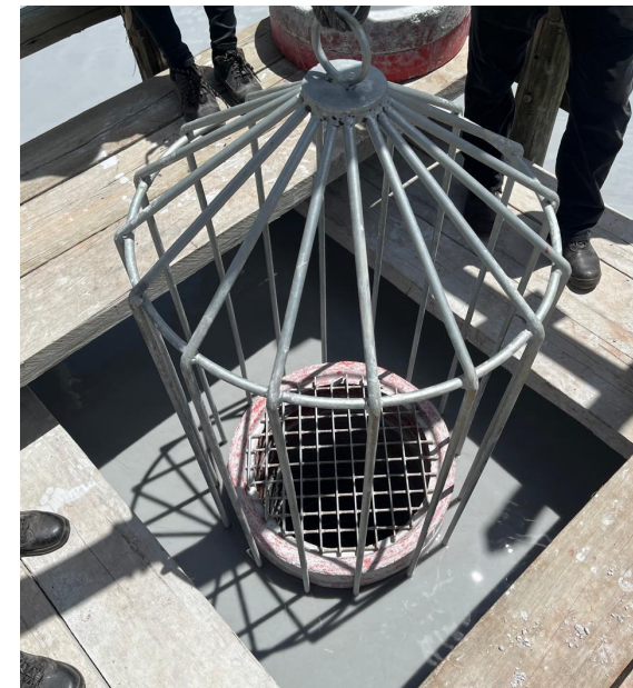
Photo: SRK archives – ringed penstock tower
