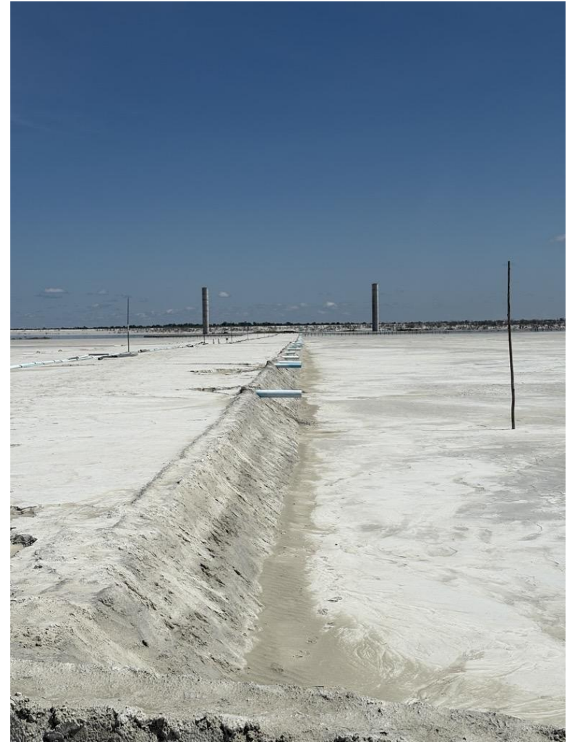
Photo: SRK archives - tailings causeway on platinum TSF
