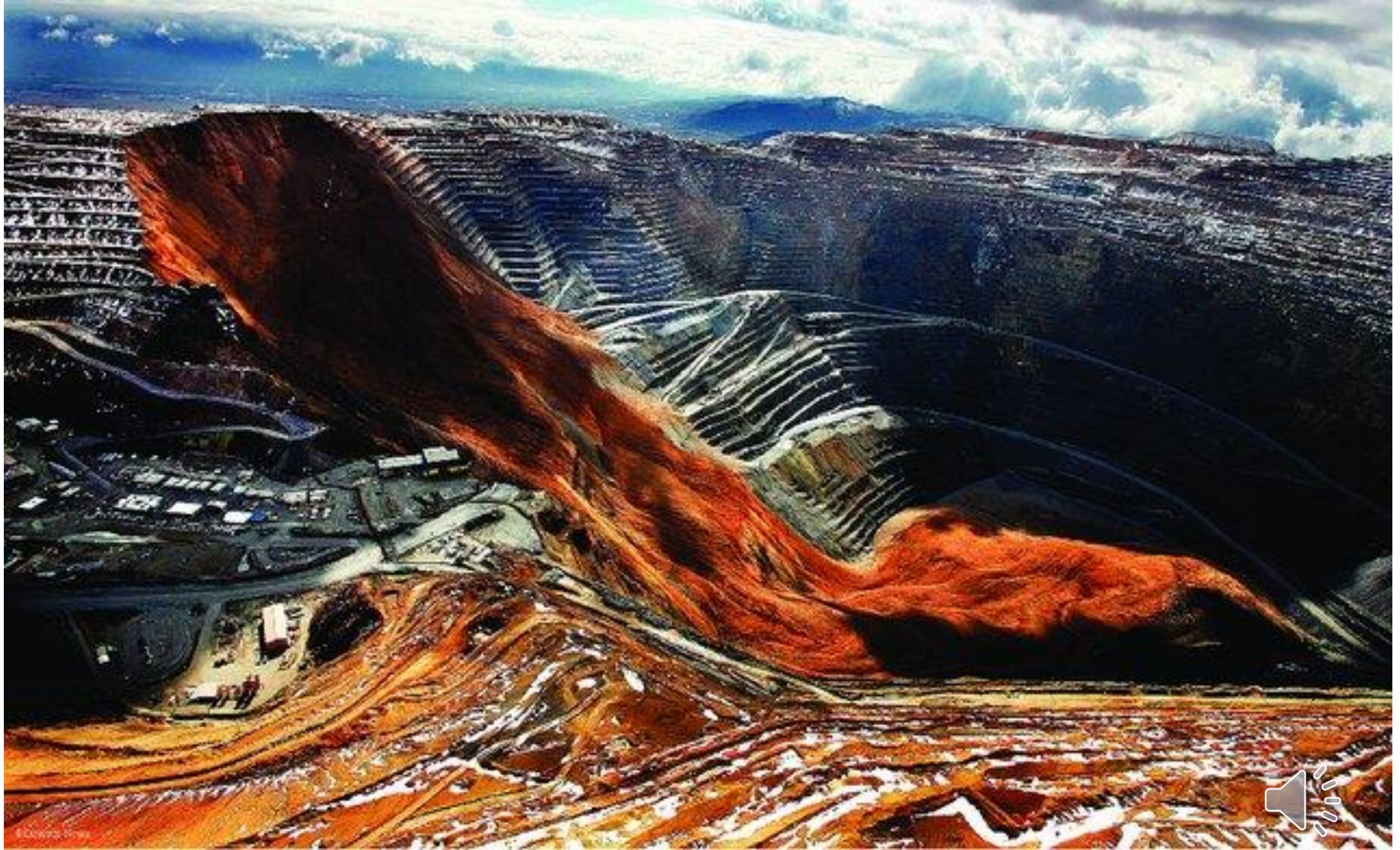
Figure 1: Slope failure. Bingham Canyon Mine. Utah / USA (Source: http://www.mining.com )
